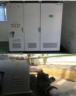
Two Cooling towers Pumps of capacity in Membrane cell I & II replaced with single pump by rationalising head with flow requirement.
